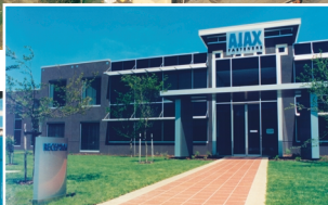
AJAX FASTENERS NEW PLANT BRAESIDE VICTORIA.
